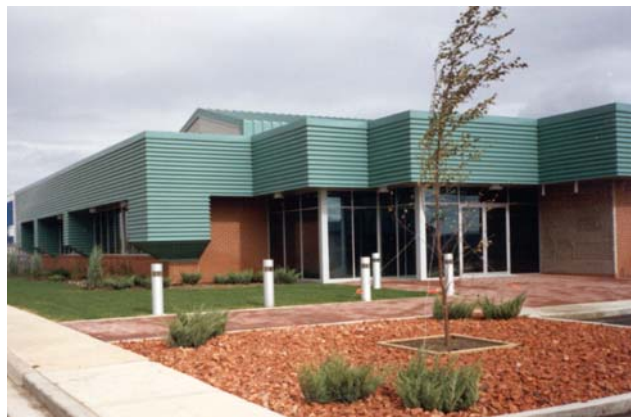
Façade at the front of the SLS HQ
